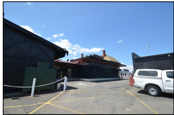
Figure 28: View from commercial car park onto south façade of heritage-item, primarily obstructed by side extension.
