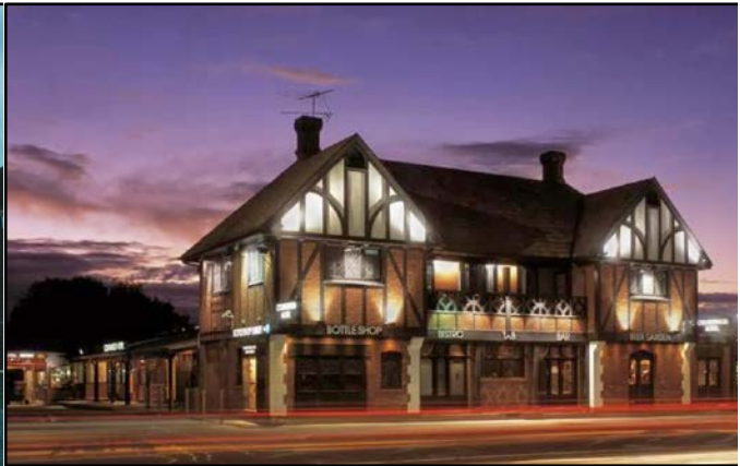
Figure 14: Primary façade of the Collingwood Hotel as it is today (Source: Google Maps and Photos, available at: https://www.google.com.au/maps/ , accessed 09.01.15)
