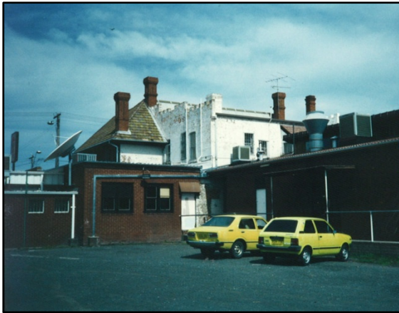
Figure 13: Colour photograph of the rear of Collingwood Hotel (west façade) as it appeared in 1991 (Source: National Library of Australia: available at: http://trove.nla.gov.au/ , accessed 09.01.15)
