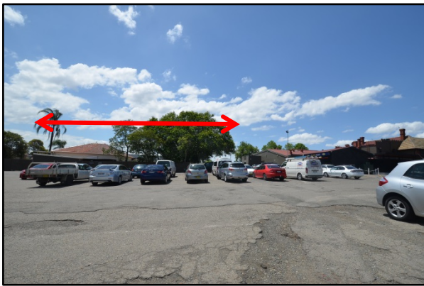
Figure 27: View from car park on site of the heritage item onto south boundary of the rear portion of the subject site indicated by the red arrows. The Collingwood Inn Hotel in located on the right hand-side. Views from the car park are given onto areas of less significance (rear and side extensions).
