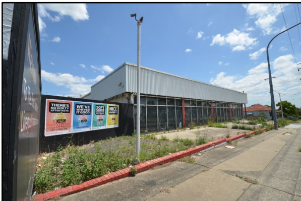
Figure 23: Existing adjacent commercial building to the north-west of the subject site.
